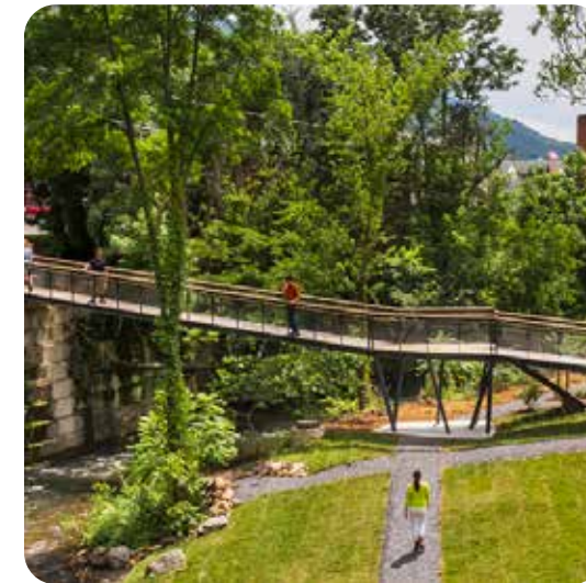
Signature pedestrian bridge
